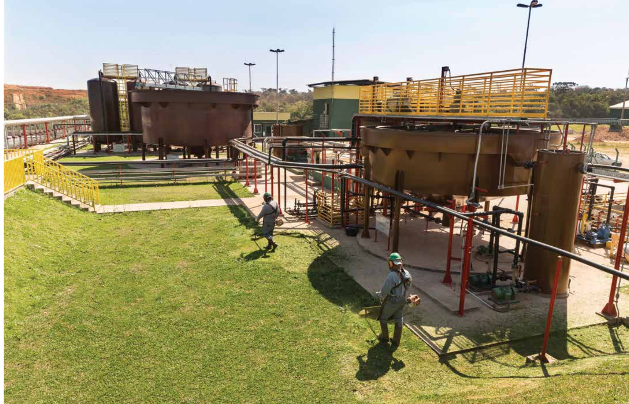
Effluent Treatment Plant: combined division results helped to balance Group financial performance
