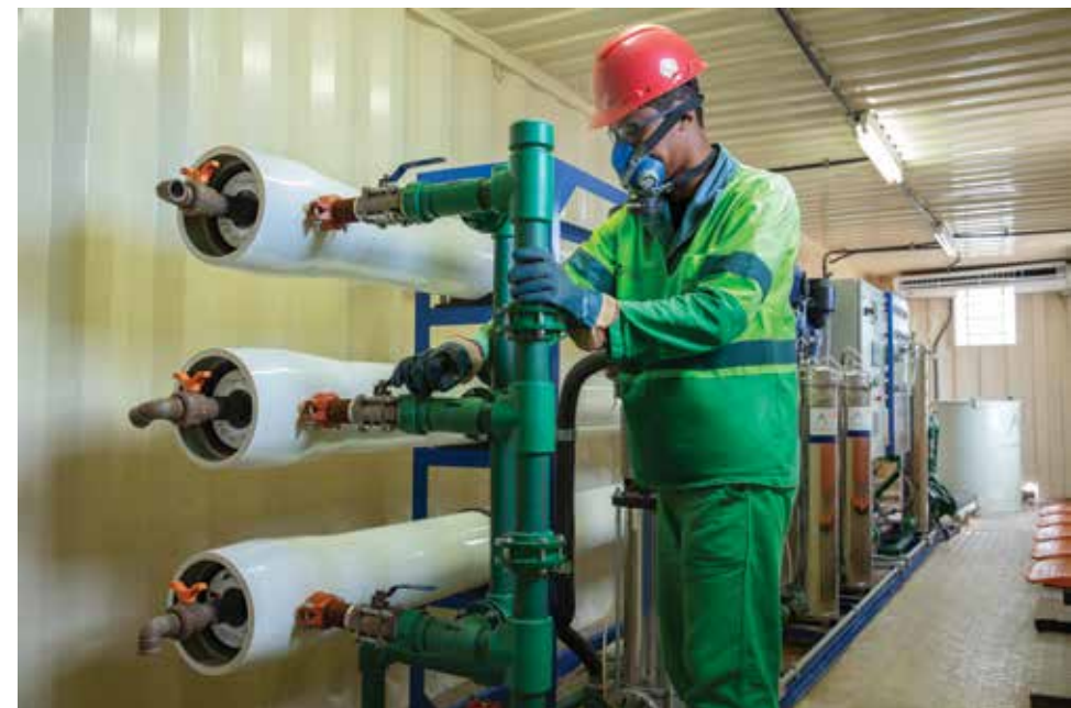
An employee working at the effluent treatment plant in Maceió (AL)
